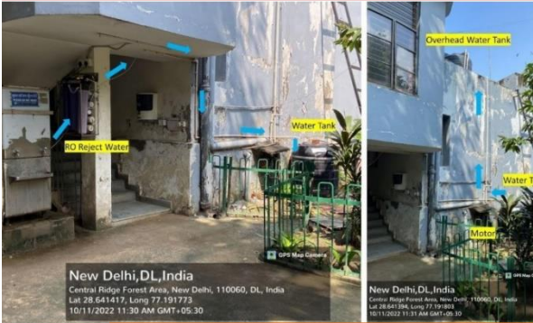
Recycling of RO wastewater
